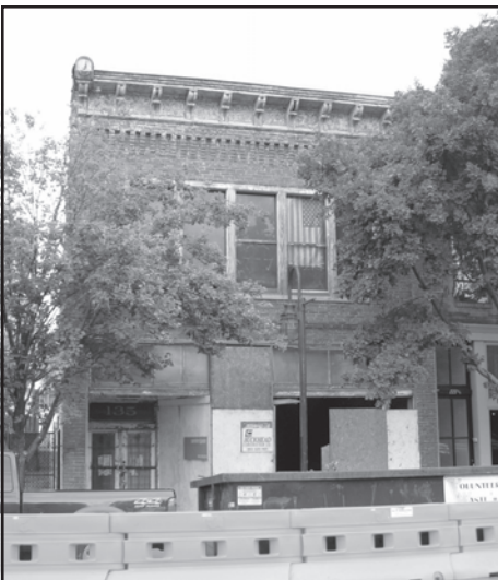
Street view of 135 Central Ave., Knoxville, Tenn. during renovation and digging.
