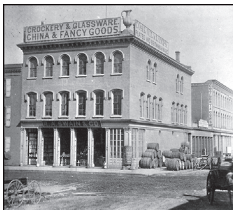
Figure 8: R.A. Swain building, San Francisco.
