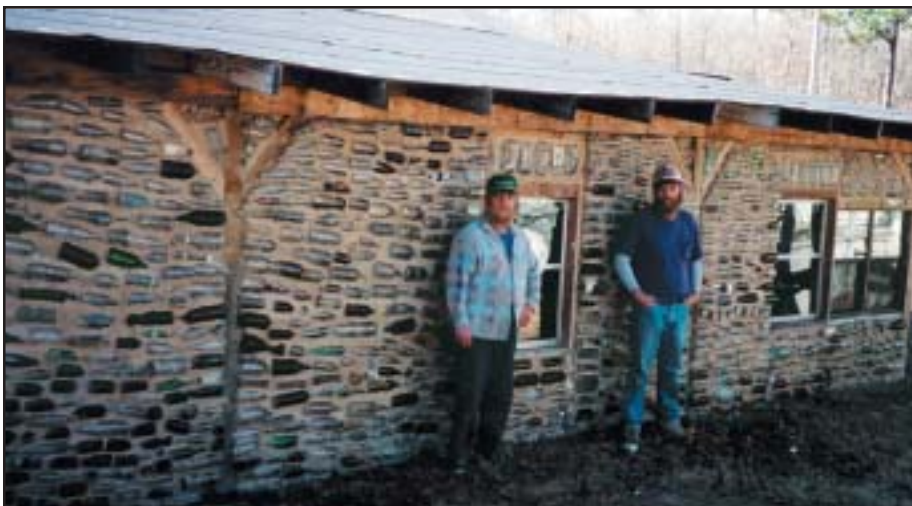
Aaron (left) and Hank Currence of Windsor in Aiken County, South Carolina have been digging and selling old bottles for several years. They dug so many, they ran out of storage room, so they decided to erect a building and use bottles instead of bricks. Mixing the mortar themselves, they'd put a layer down and then a layer of bottles, then another mortar base and then another layer of bottles. It took them four months to finish the 50-foot-long, 30-foot-wide structure. It's a joy for them to inside the building during sunrises and sunsets, peak times for the sunlight to shine through the walls.
