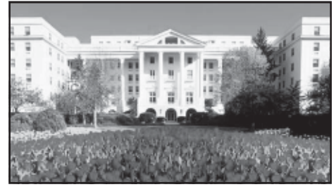
Main Street entrance to the Greenbrier.
