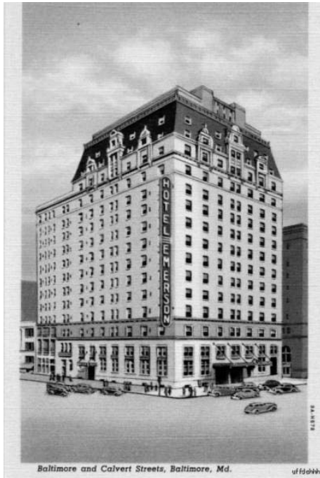
Figure 14 - New Emerson Hotel (1936) in Baltimore, Maryland
