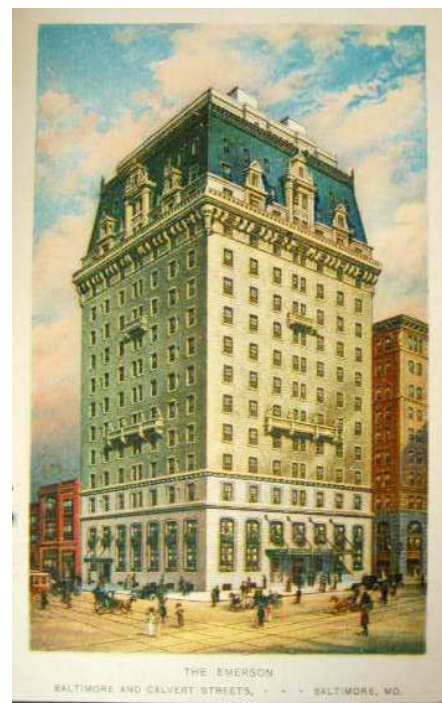
Figure 13 - Emerson Hotel (1910 view) Baltimore, Maryland
