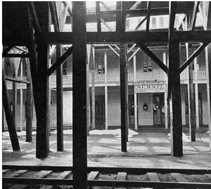
Passengers disembarking at Summit Station were presented with a forest of posts that supported the huge roof of the snow shed. From this point the Summit Soda Springs were another 15 miles by horse. (8)
