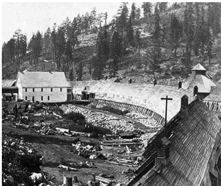
The newly constructed Summit Station with the Summit House on the left. Massive snow sheds were necessary to keep from paralyzing the movement of trains during the winter months. Construction of the C.P.R.R. to this point allowed for the cost effective harvesting of ice. This photo was probably taken no later than 1870 since the denuded landscape shows no sign of revegetation. (6)
