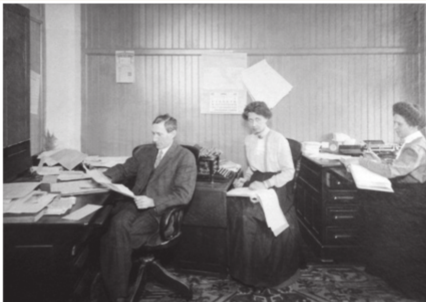
Fig. 7: Main Office at 126 Chambers Street, New York Photograph taken in April, 1901
