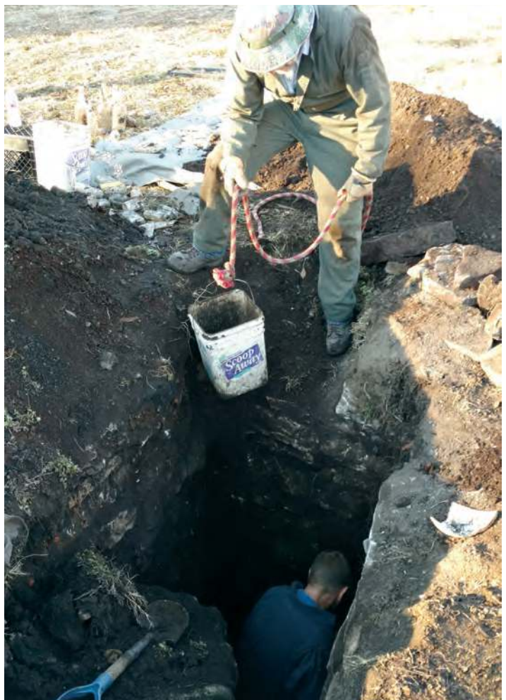
Kenny digging while Ed pulls buckets
