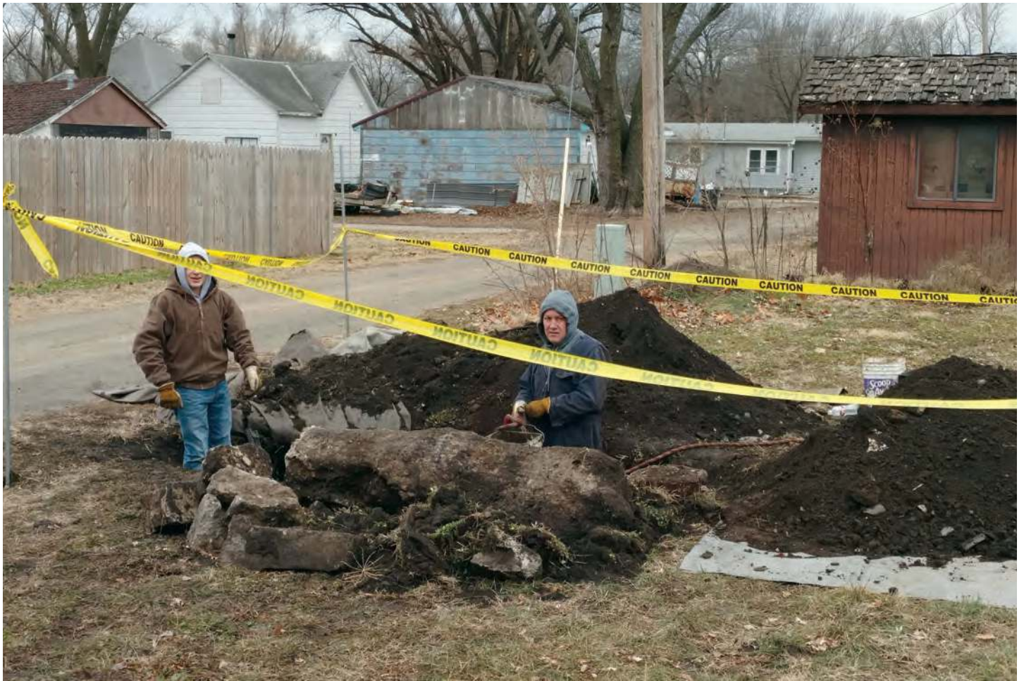
Caution tape was strung around the hole to keep the hole safe from people walking through the lot.
