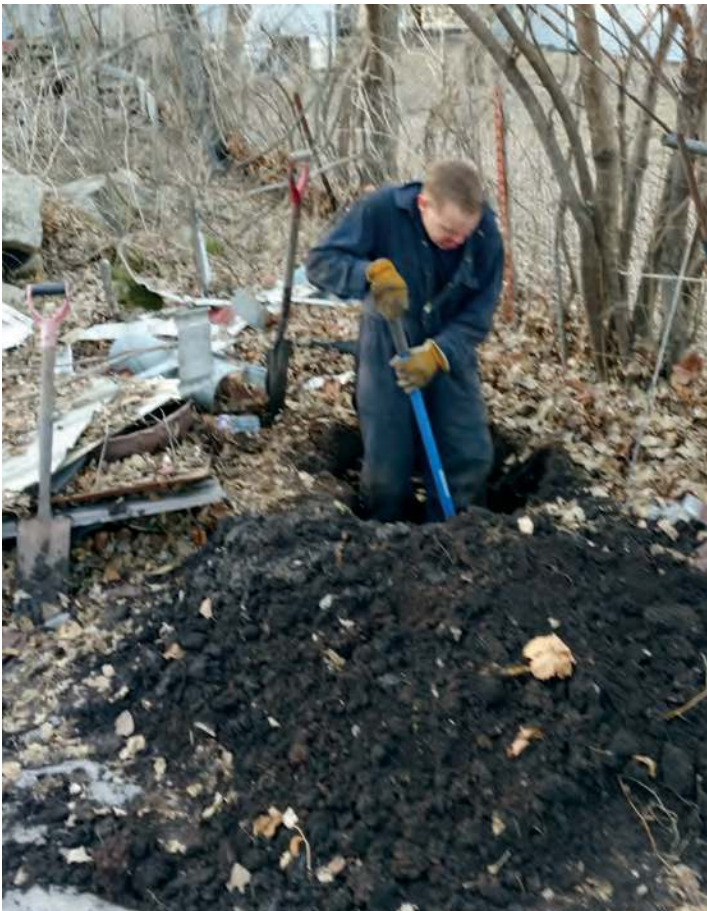
Kenny digging the "sloppy" hole at the Iowa Hotel.
