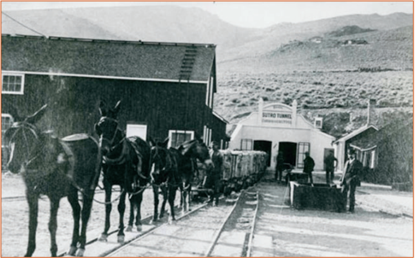
Original Photo of the Sutro Tunnel
