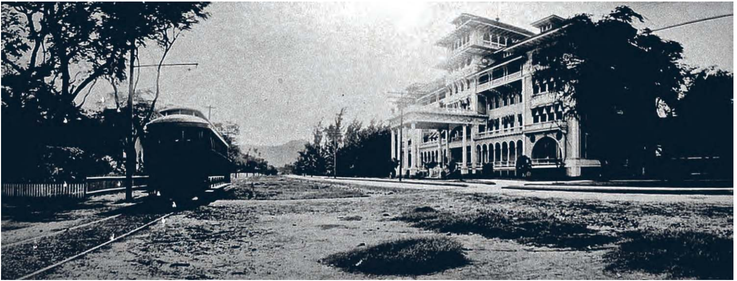
Fig.12: The newly finished Moana Hotel with a tramway in front taking visitors to nearby Diamond Head.
